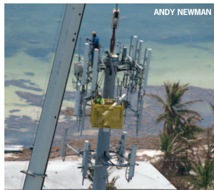
Technicians repair cellular antennas.
