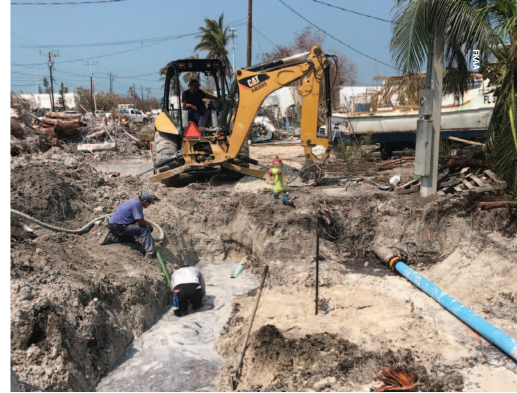
A Florida Keys Aqueduct Authority crew repairs a water line break.
